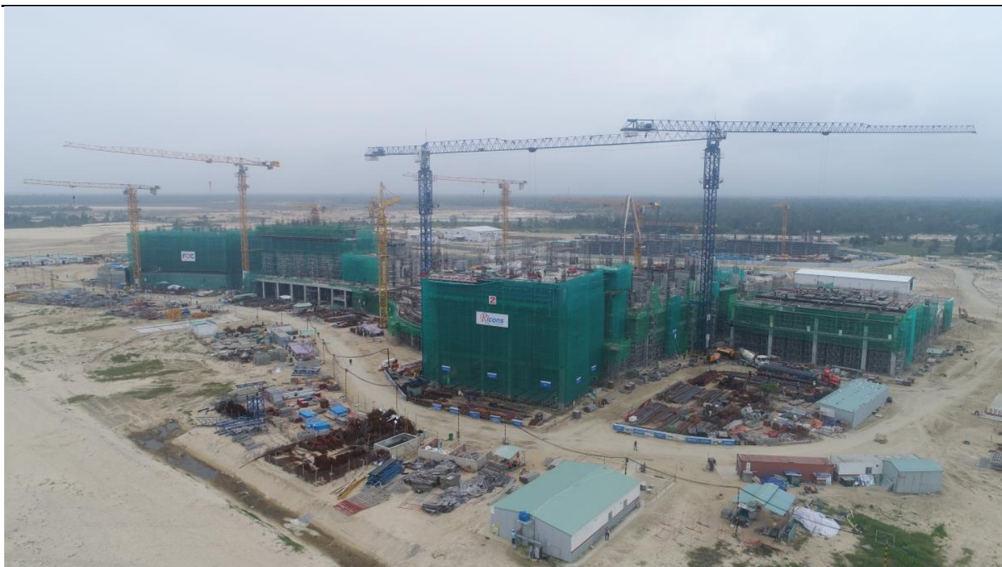
Figure 1: Hoiana construction progress (as of January 2018)
